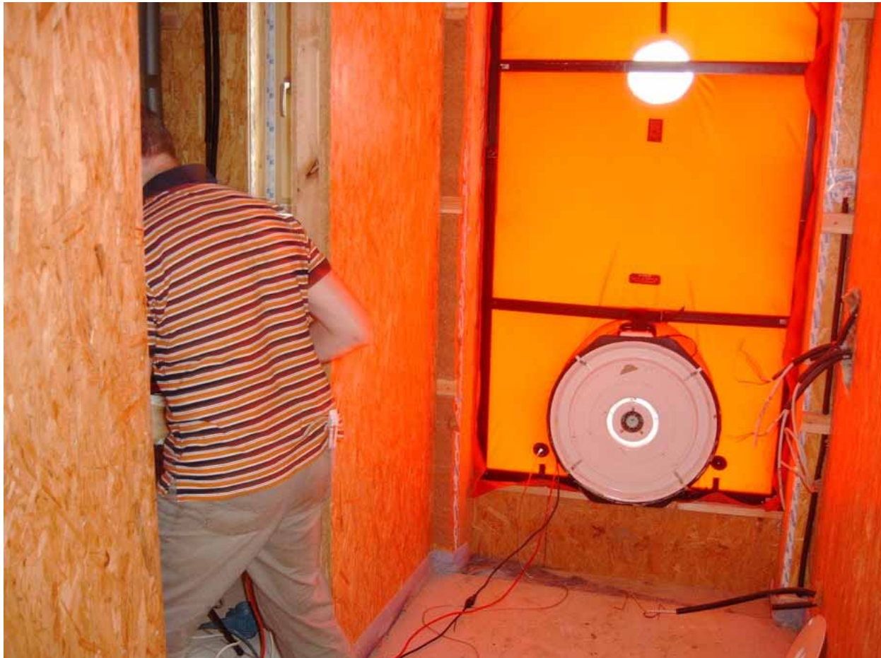
Fig. 9: Pressurization test “Blower-Door-Test” - Friedl, Architect ©
