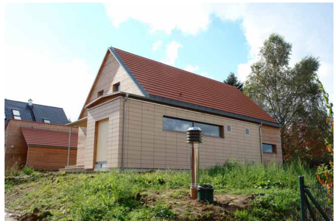
Fresh air suction tower
