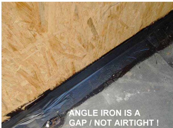
Fig. 10: Airtightness - Friedl, Architect ©
